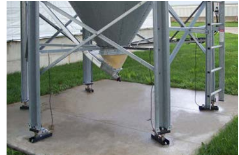
Load Cells handle up to 10,000 pounds (4,500 kg) per feed bin leg.
