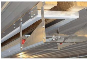
TURBO® Inlets (above) running the length of cage rows provide a controlled stream of fresh air in two directions as part of the TURBO HOUSE® System.
