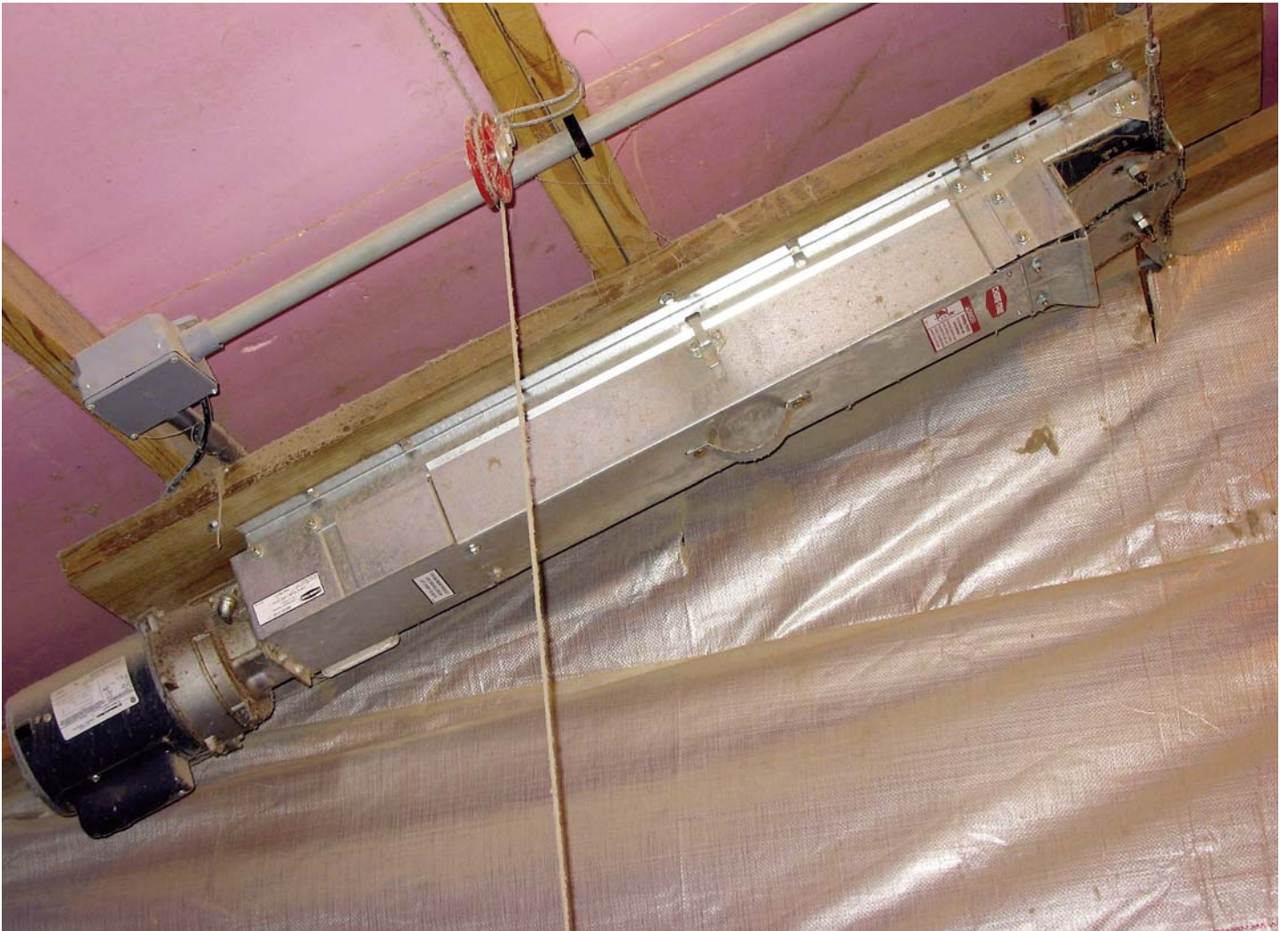
Chain-type linear drive
