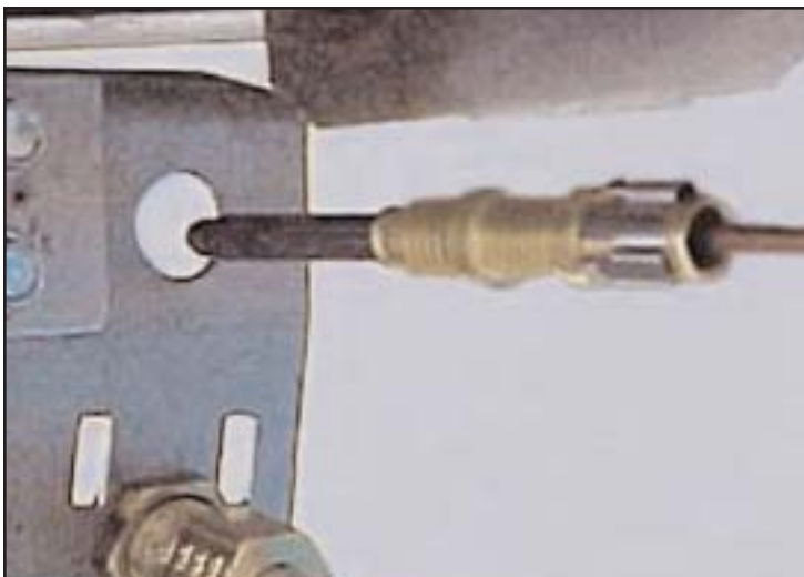
(14) Insert THERMOCOUPLE into the PILOT BRACKET .
