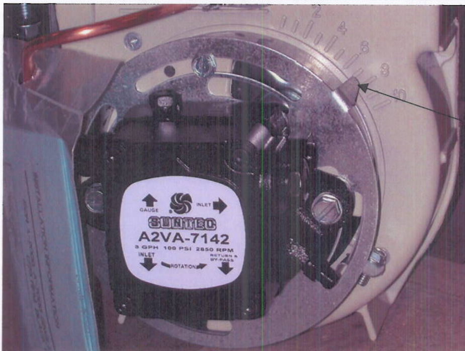
Air Shutter indicator (Beckett burner)
