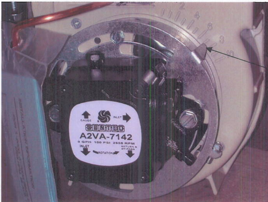
Air Shutter indicator (Beckett burner)
