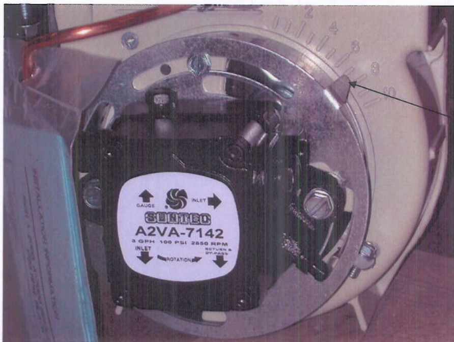
Air Shutter indicator (Beckett burner)
