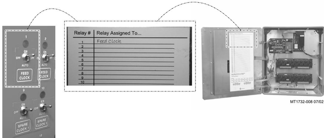
**Figure 41. Relay Assignments**
