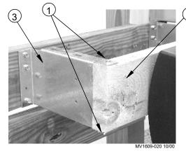
Figure 7. Bottom Bracket Connection
