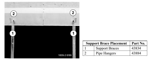
Figure 10. Close-up View of Support Brace Installation
