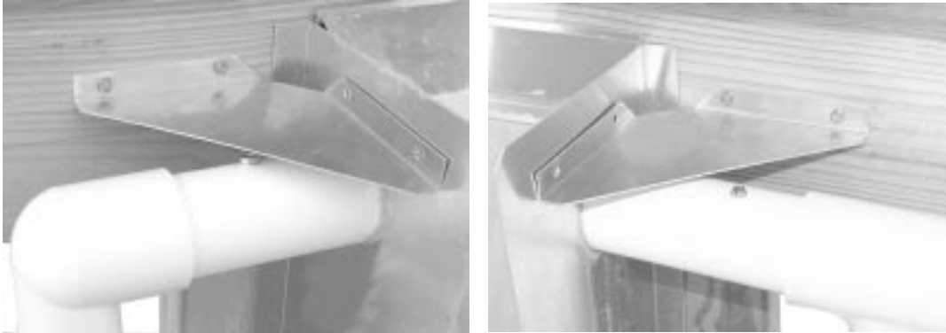
Figure 14. End Panel Support Installation
