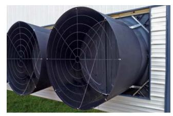
Chore-Time's 57-inch EnduraMax<sup>™</sup> Direct-Drive Fan with HYFLO<sup>®</sup> Shutters features a variable speed motor to help maximize energy efficiency.
