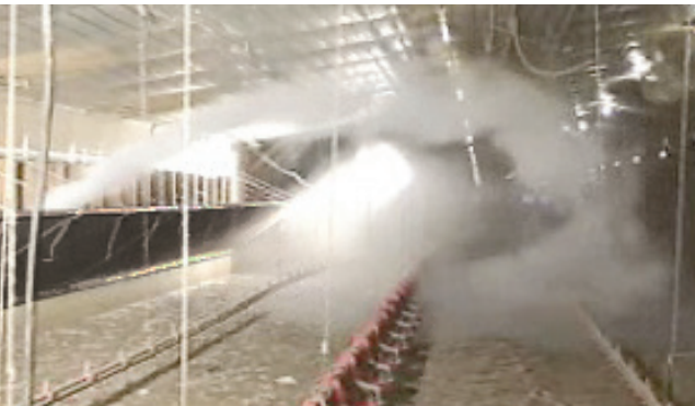
Air shoots upward and then swirls down and around from center of house for outstanding air mixing.
