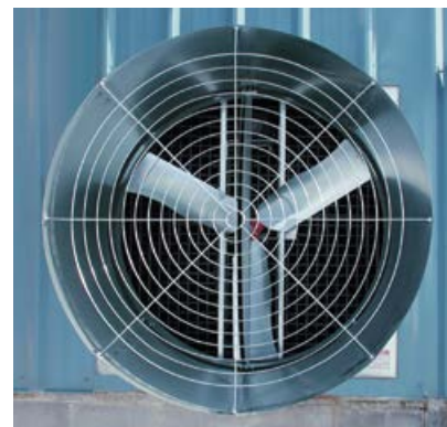
HYFLO® Shutter doors are pushed open as air is exhausted when fan operates.
